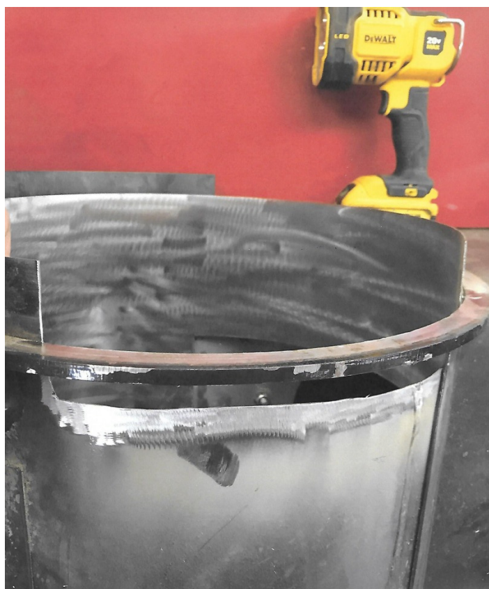
USE PART OF THE 2 3/4 INCH RING SUPPLIED IF NEED PUT IN PLACE BEFORE INSTALLAING VRTICAL LINER
